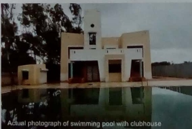
Actual photograph of swimming pool with clubhouse
