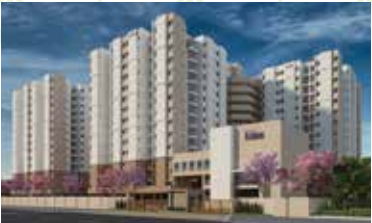
ASHRAYA Bengaluru - Mysuru Expressway, Bidadi
