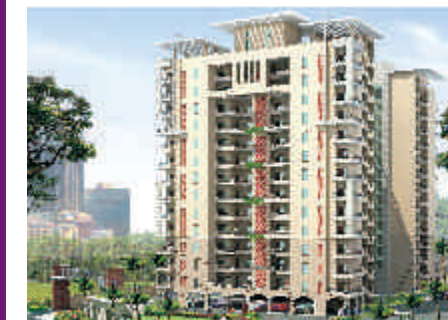
ImpressionsPlus, Rajnagar Extn., Ghaziabad (Under Construction)
