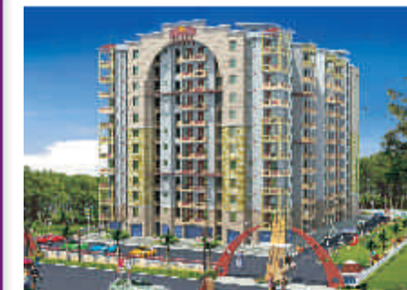
Impressions58, Rajnagar Extn., Ghaziabad (Under Construction)
