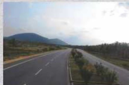
ROADS & HIGHWAYS PROJECTS
