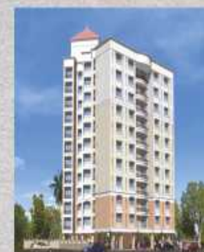
GANGA TOWER CHEMBUR
