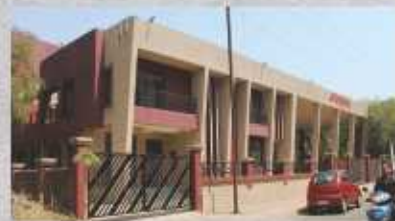
FIRE STATION - KOPERKHAIRANE
