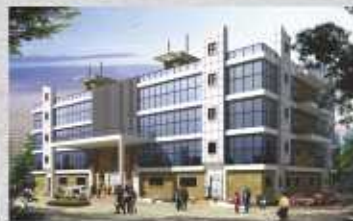
MCH HOSPITAL - BELAPUR
