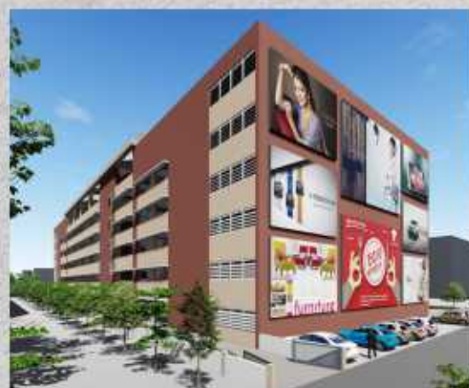
PARKING TOWER BUILDING CBD BELAPUR
