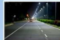
PWD 6 Lane Road
