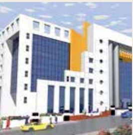
SILICON PLAZA PUNE
