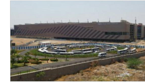
IT Park Adibatla (TCS)
