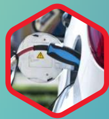
VEHICLE CHARGING POINT
