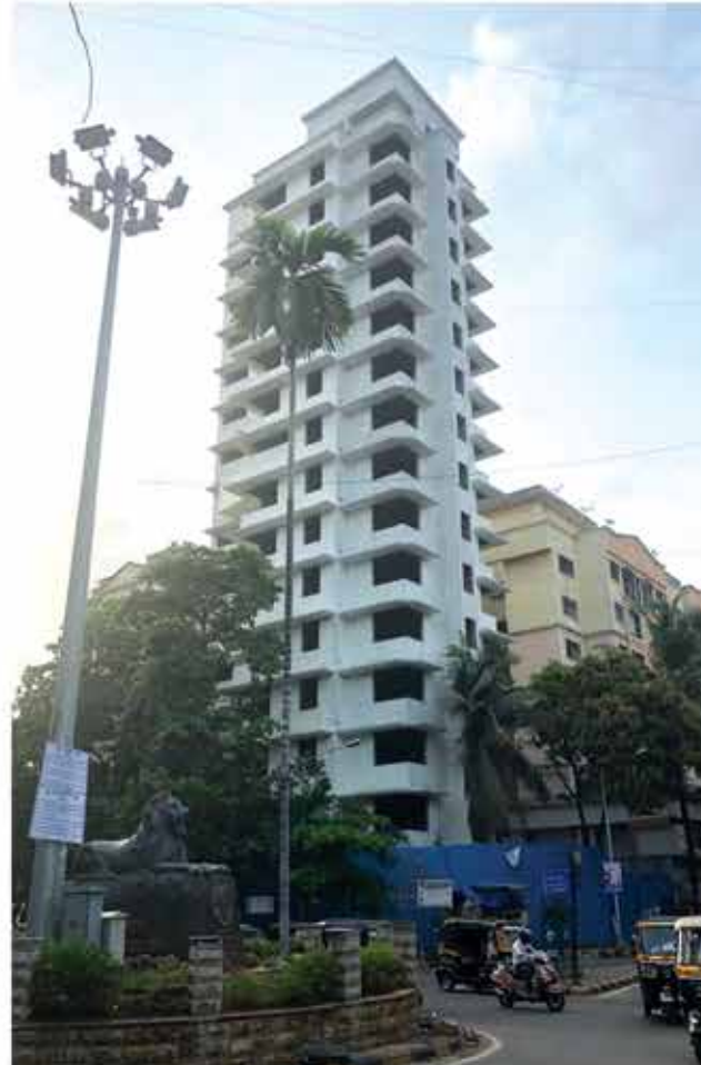
Riddhi Siddhi Tower, Tilak Nagar, Chembur.
