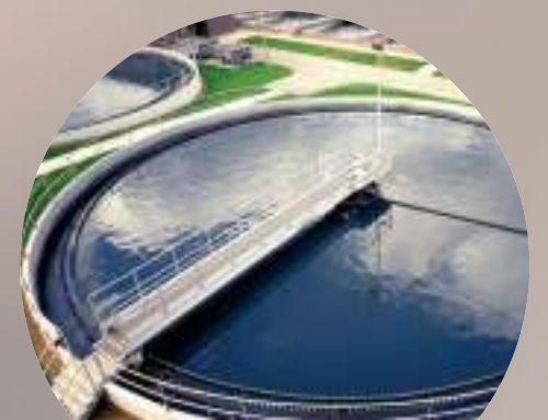
Sewerage Treatment Plant (STP)
