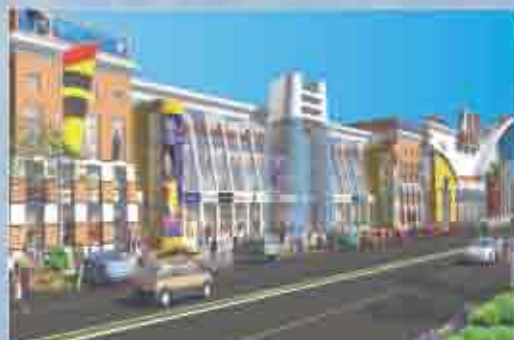
Aditya City Centre, Indirapuram
