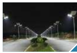
INTERNAL RCC ROAD WITH STREET LIGHT
