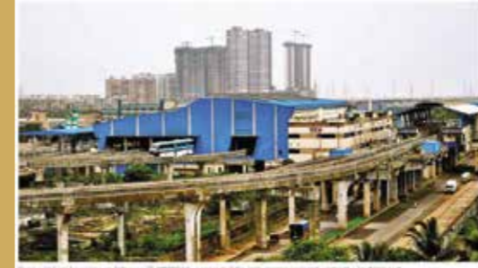
Mumbai Metropolitan Region Development Authority (MMRDA) has started a plan to undertake Transport Oriented Development (TOD) of land around the existing monorail depot situated in Wadala.
