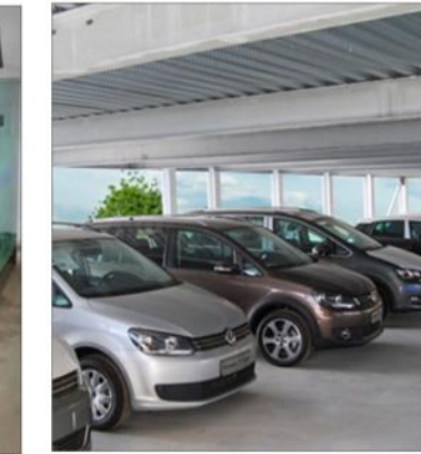
Covered Car Parking
