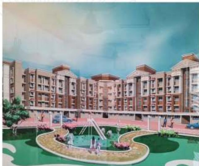
GHANSHYAM PARK RESIDENTIAL BUILDING
