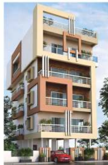
GHANSHYAM PALACE RESIDENTIAL BUILDING VASAI (W)
