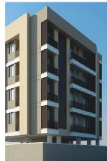
GHANSHYAM VINDHYAGIRI APARTMENT RESIDENTIAL BUILDING VIRAR (E)
