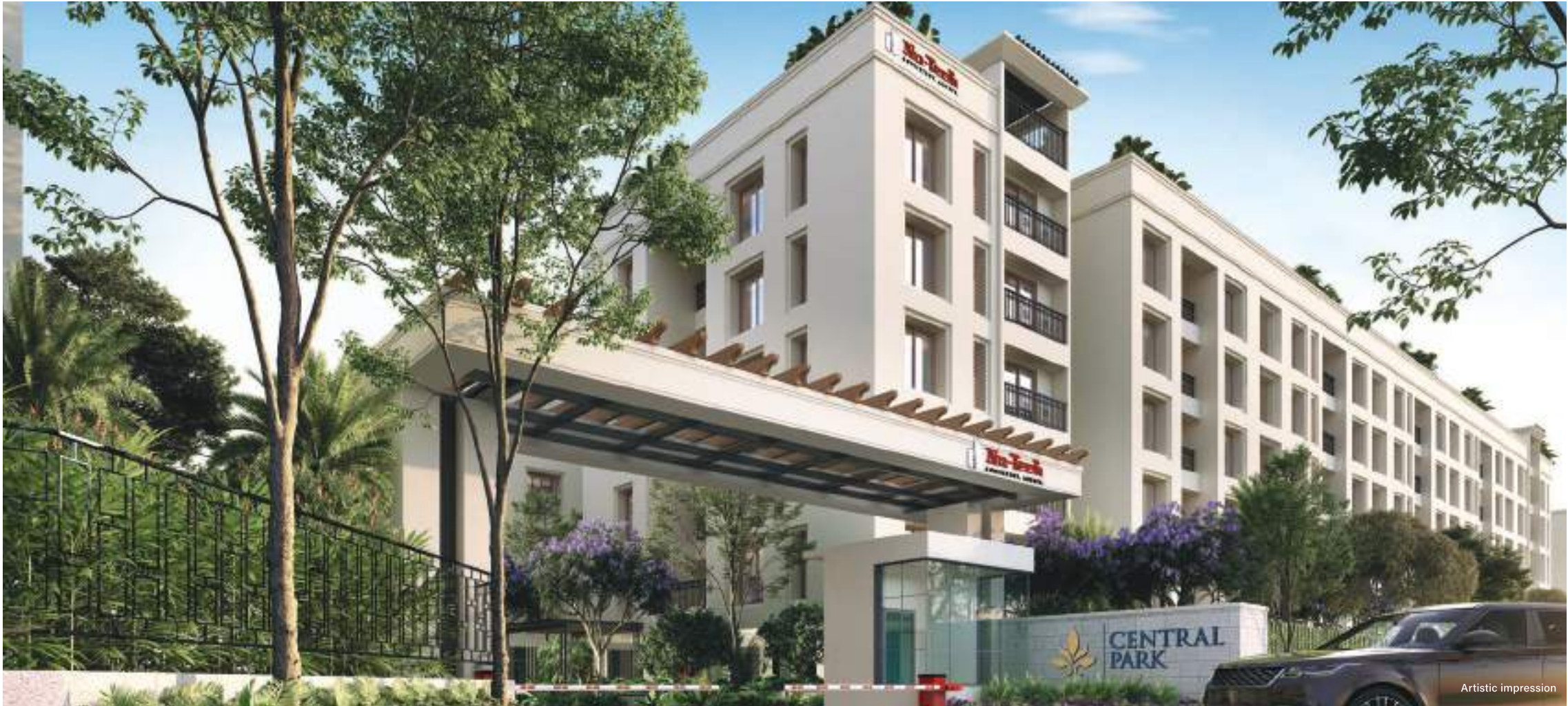
Flood-resistant homes that survive every weather condition.
