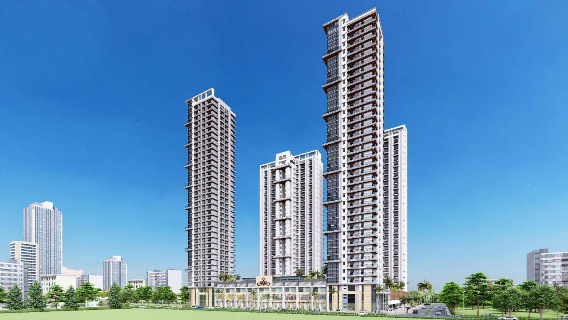
'REGENCY PALMS', PROPOSED COMMERCIAL & RESIDENTIAL BUILDING, PLOT NO. R/3A, SECTOR-14 A, NERUL, NAVI MUMBAI.
