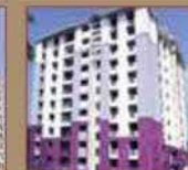
PALACE HEIGHTS Kottaram Road
