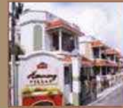
HARMONY-VILLAS Sakthan Thampuran Nagar
