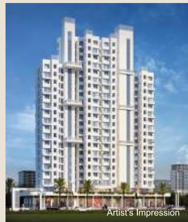
ONGOING PARTH SKYONE DOMBIVLI - EAST
