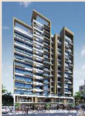
COMPLETED PARTH MAGNUS SANPADA, NAVI MUMBAI
