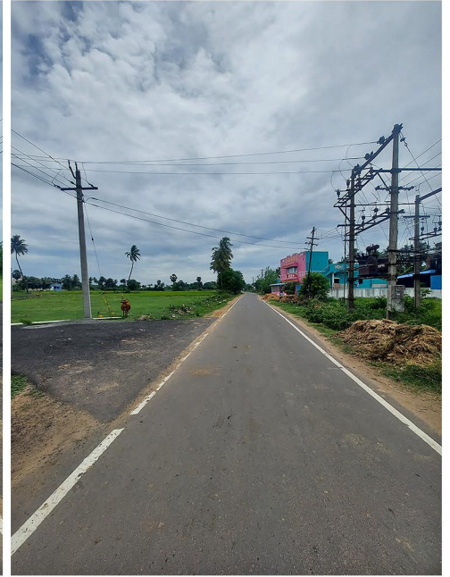
Road View from East
