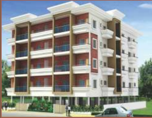
GR GREENS @ Chunchaghatta Main Road (Completed)
