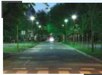
RCC Roads with Paving & Street Lights
