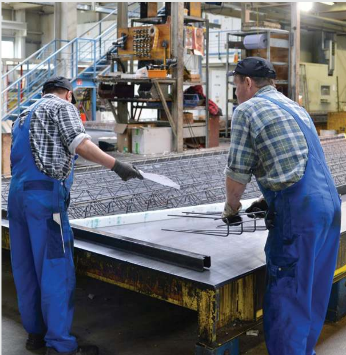
Precast Facility 73,000 sq. ft. (9,290.30 sq. m.)
