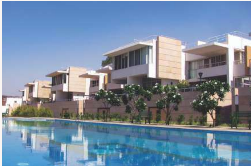
Rohan Madhuban, Bavdhan, Pune
