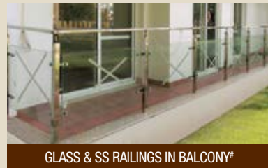
GLASS & SS RAILINGS IN BALCONY*
