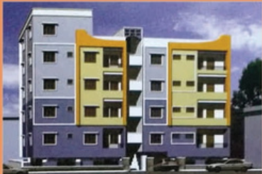
TIRUMALA APARTMENTS, BALAJI HILLS
