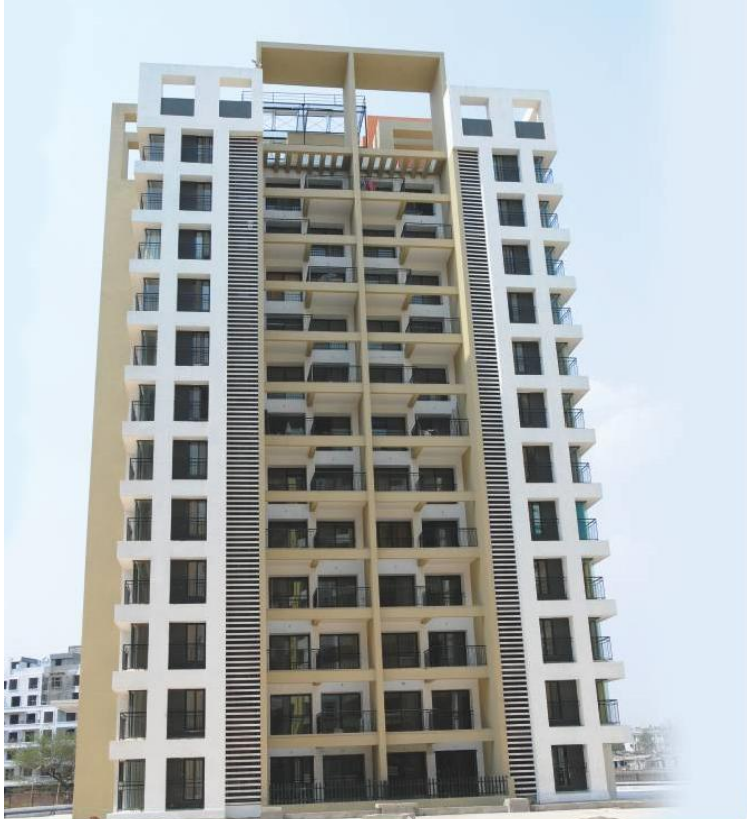
Malpani Greens at Wakad, Pune
