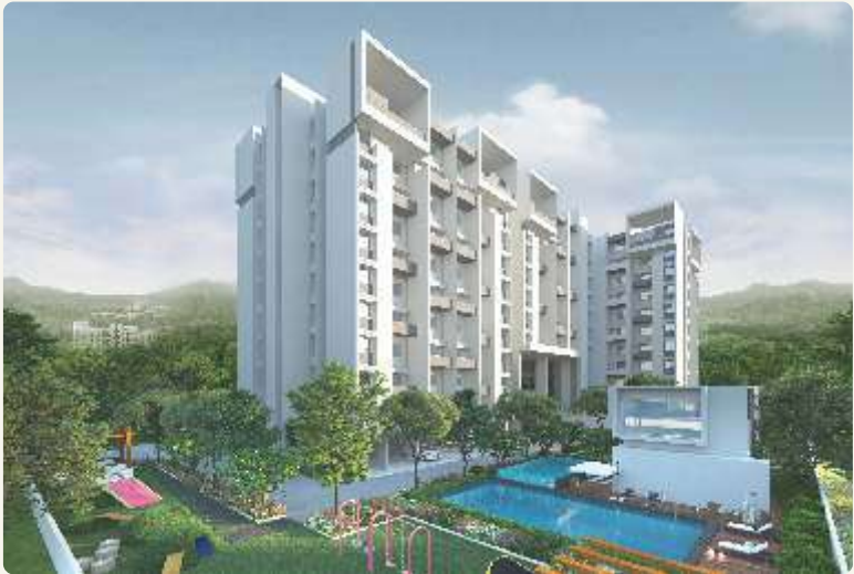
Rohan Ipsita, Hinjawadi Phase-1, Pune.
