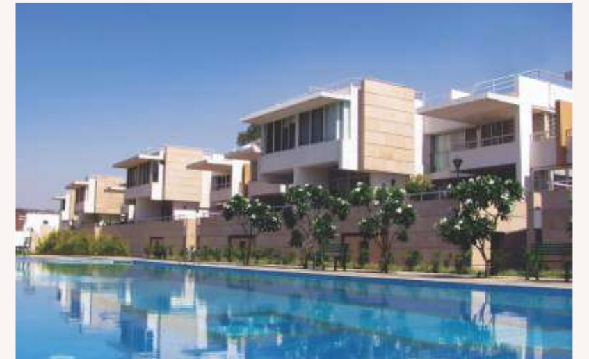
Rohan Madhuban, Bavdhan, Pune
