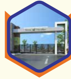
MAIN ENTRANCE ARCH
