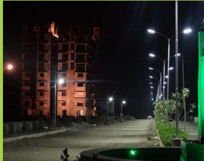
Ready Infrastructure Of Crystal city
