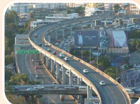
ELEVATED ROAD UPTO DELHI
