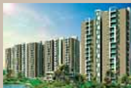
APARNA HILLPARK LAKEBREEZE (Work in progress) 943 Loveneests, Miyapur, Chandanagar
