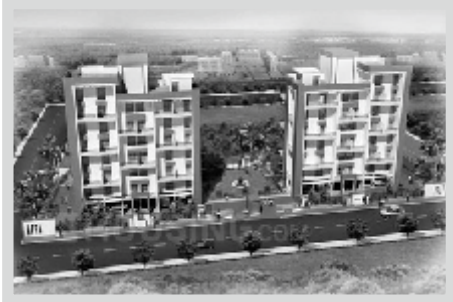
Fortune Mirador Baner, Pune
