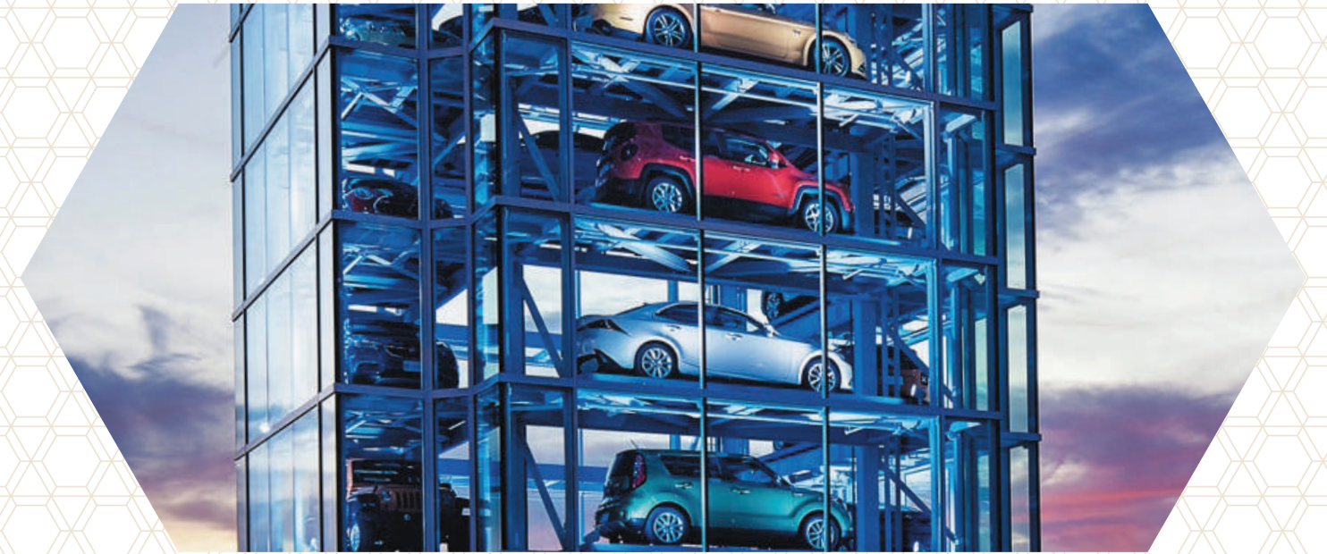
Multilevel Vehicle Parking Tower
