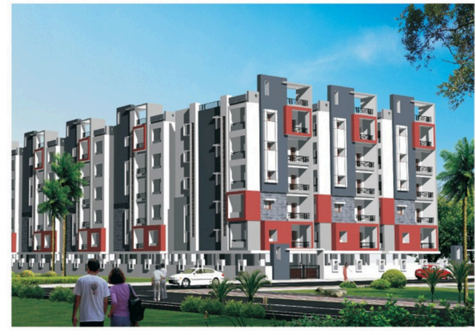
Sanjanamalathi Residential Complex
