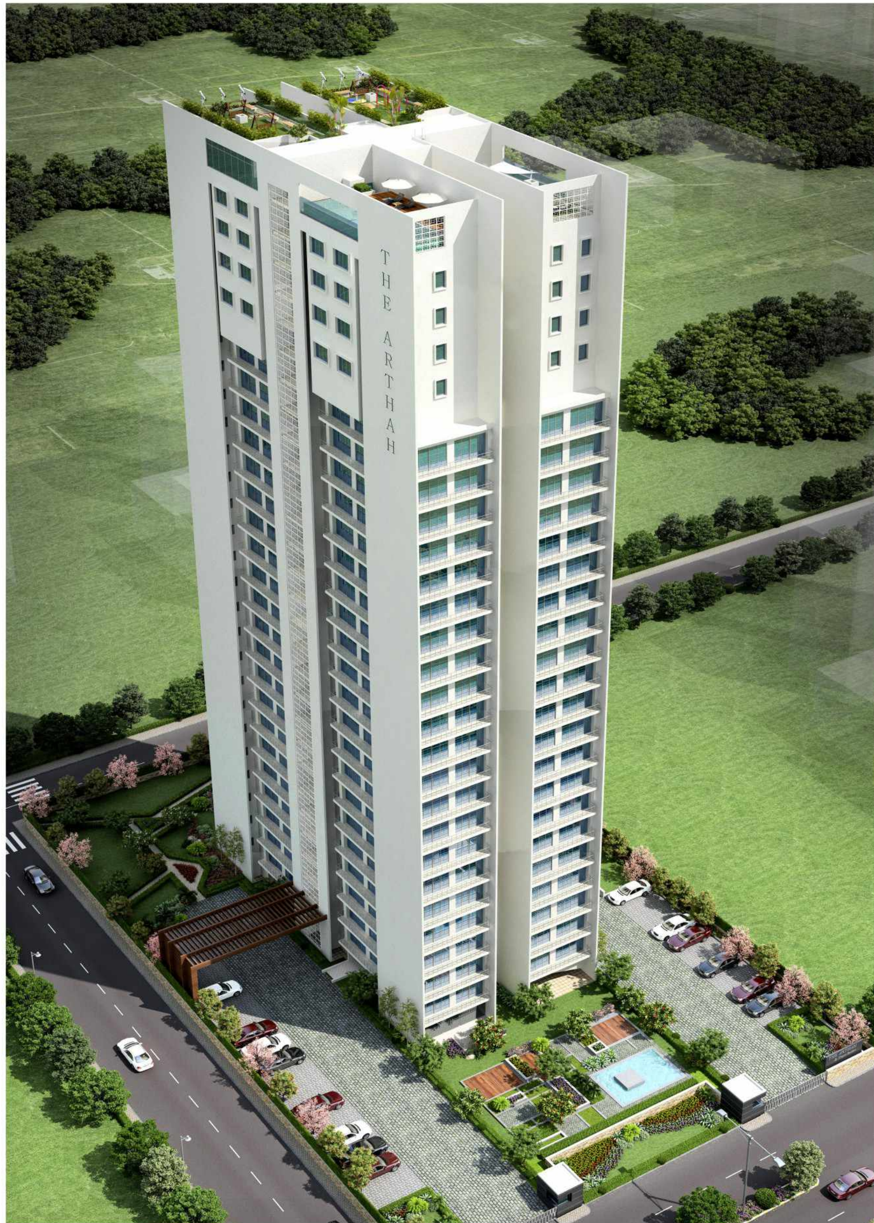
AERIAL VIEW with Roof-top Club
