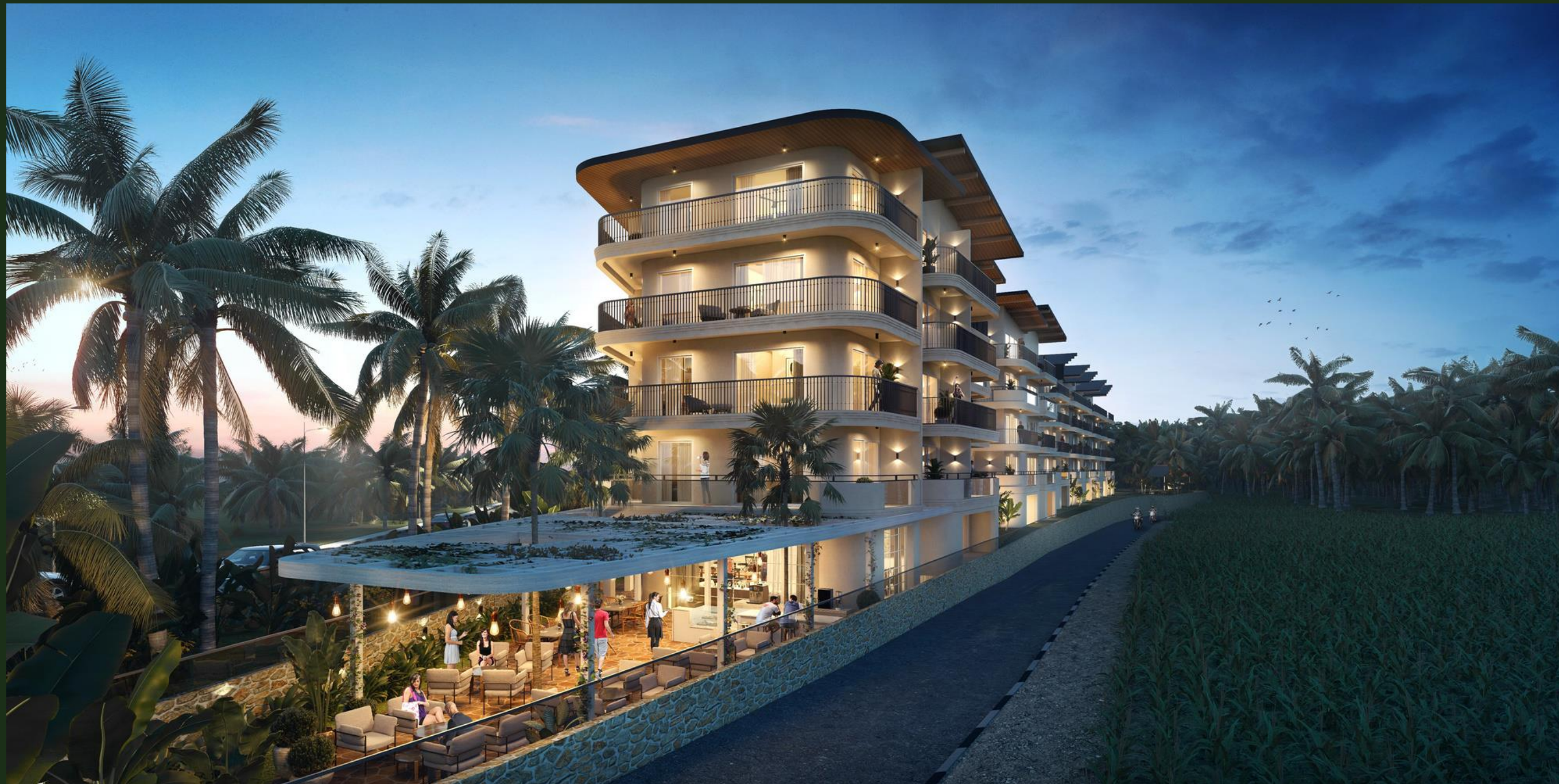
Vista Arrozal, Goa UNDER CONSTRUCTION
