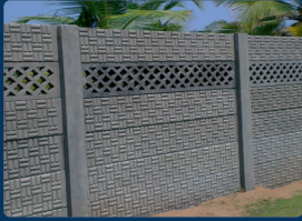
Boundarywall for Campus
