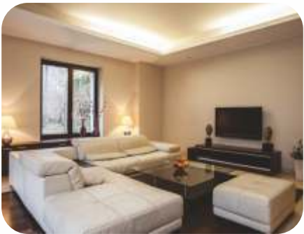
POP Ceiling in Living Room with LED Light
