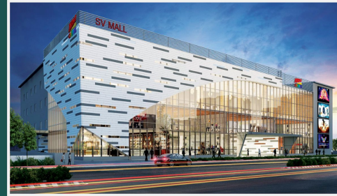
SV Mall @ Adibatla
