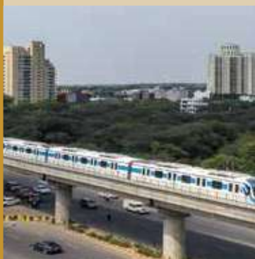
MUMBAI METRO LINE 5
