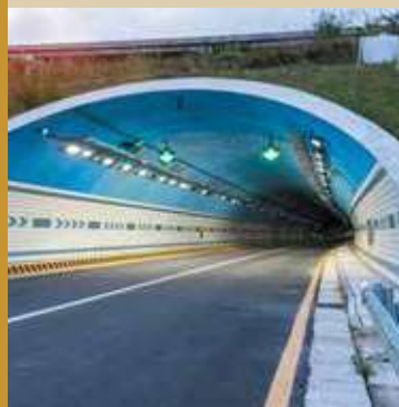
BORIVALI - THANE TUNNEL
