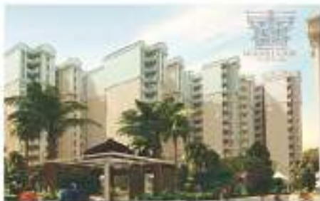
M.I. Rustle Court, Gomti Nagar, Lucknow
