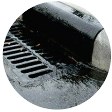
STORM WATER DRAINS
