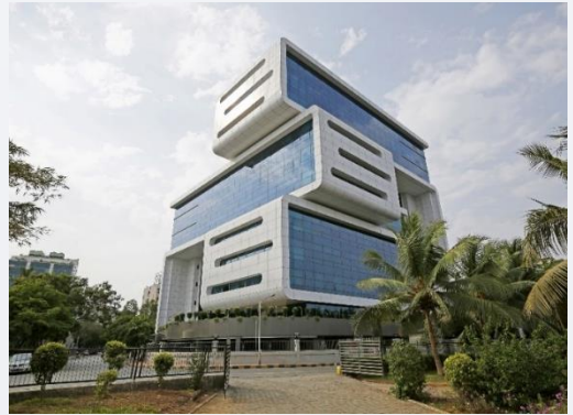
MMRDA's NEW OFFICE AT BKC, MUMBAI. (Contracting Work)
