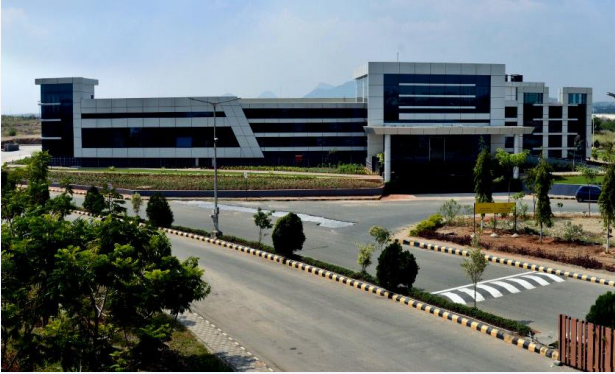
L&T ADMIN BUILDING COMPLEX , COIMBATORE. (Contracting Work)
