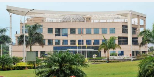
L&T ADMIN BUILDING COMPLEX, TALEGAON. (Contracting Work)
