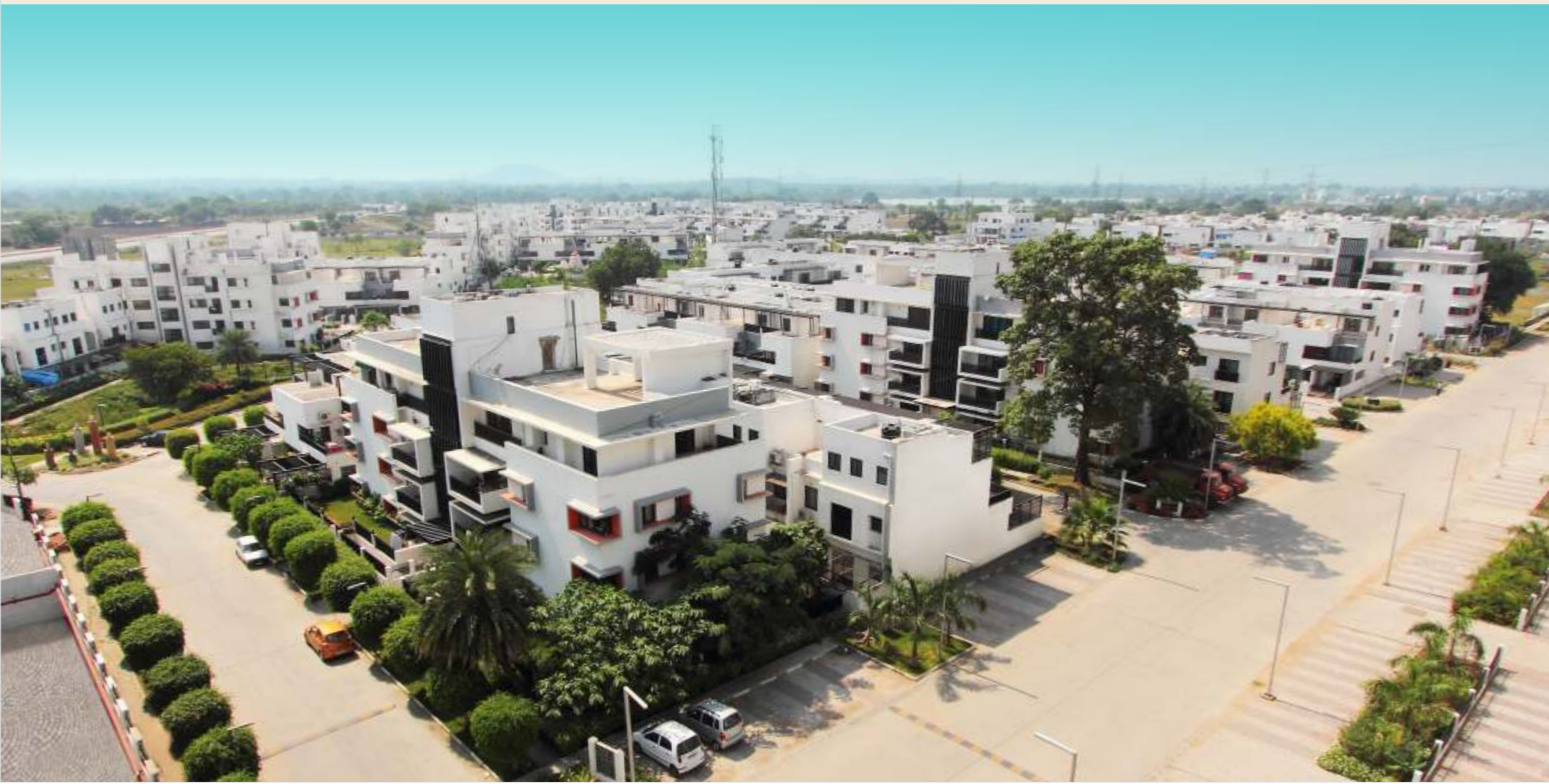
Actual Photograph of Site
