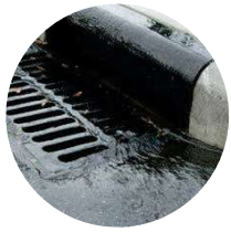
STORM WATER DRAINS
