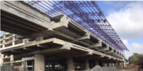
Kadugodi Metro Station
