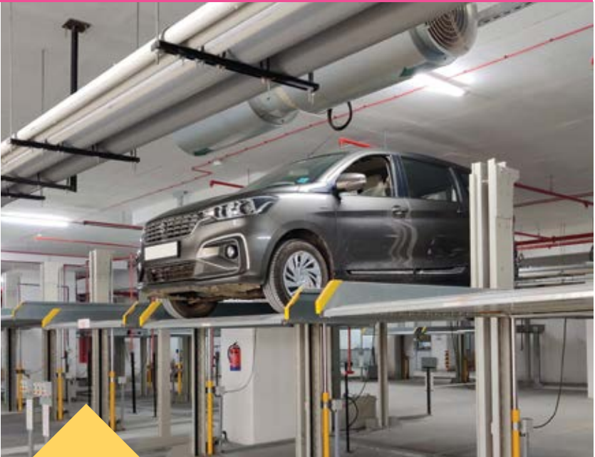
Stack parking option is provided in the basement, wherever feasible, thanks to generous slab heights.
