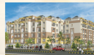
Scion Chitrakut @ CV Raman Nagar
